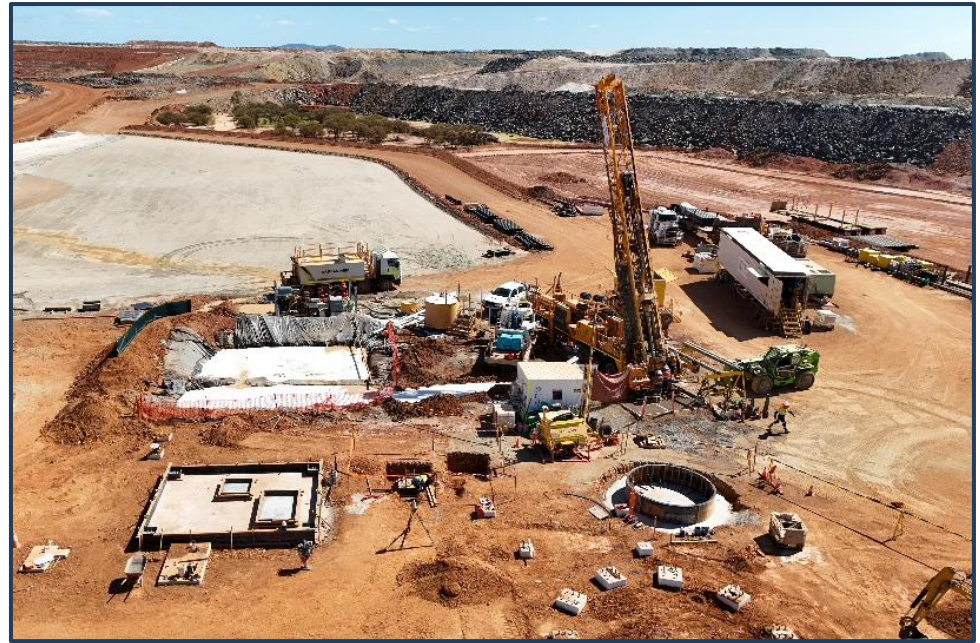
Paste plant construction
