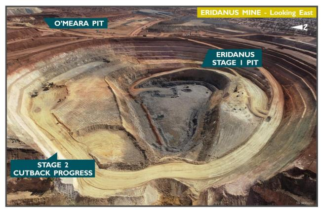
Figure 3: Eridanus pit looking East – showing Stage 2 Cutback progress
