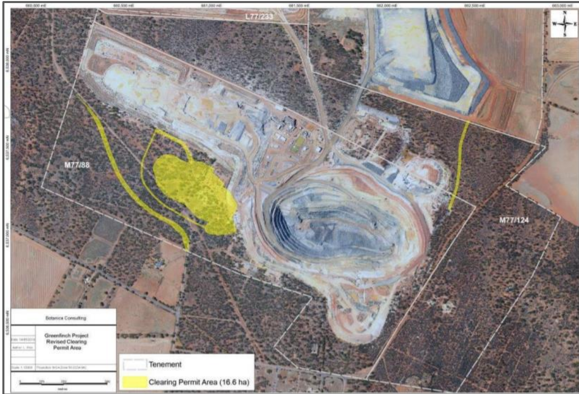
Figure 5: Edna May Stage 2 open pit and processing facility, with Greenfinch projected area highlighted in yellow
