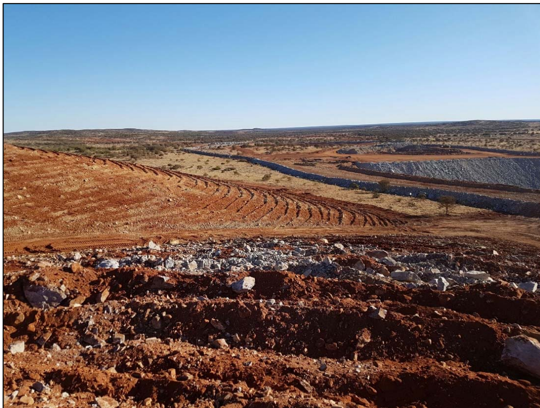
Figure 7: Yellow Aster open pit – rehabilitated waste dump & abandonment bund
