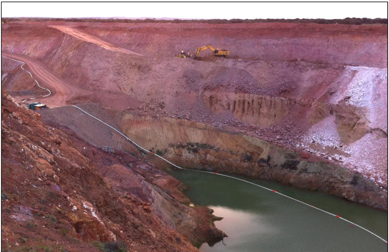
**Figure 7: Vivien pit cutback - mining and dewatering looking NE**
