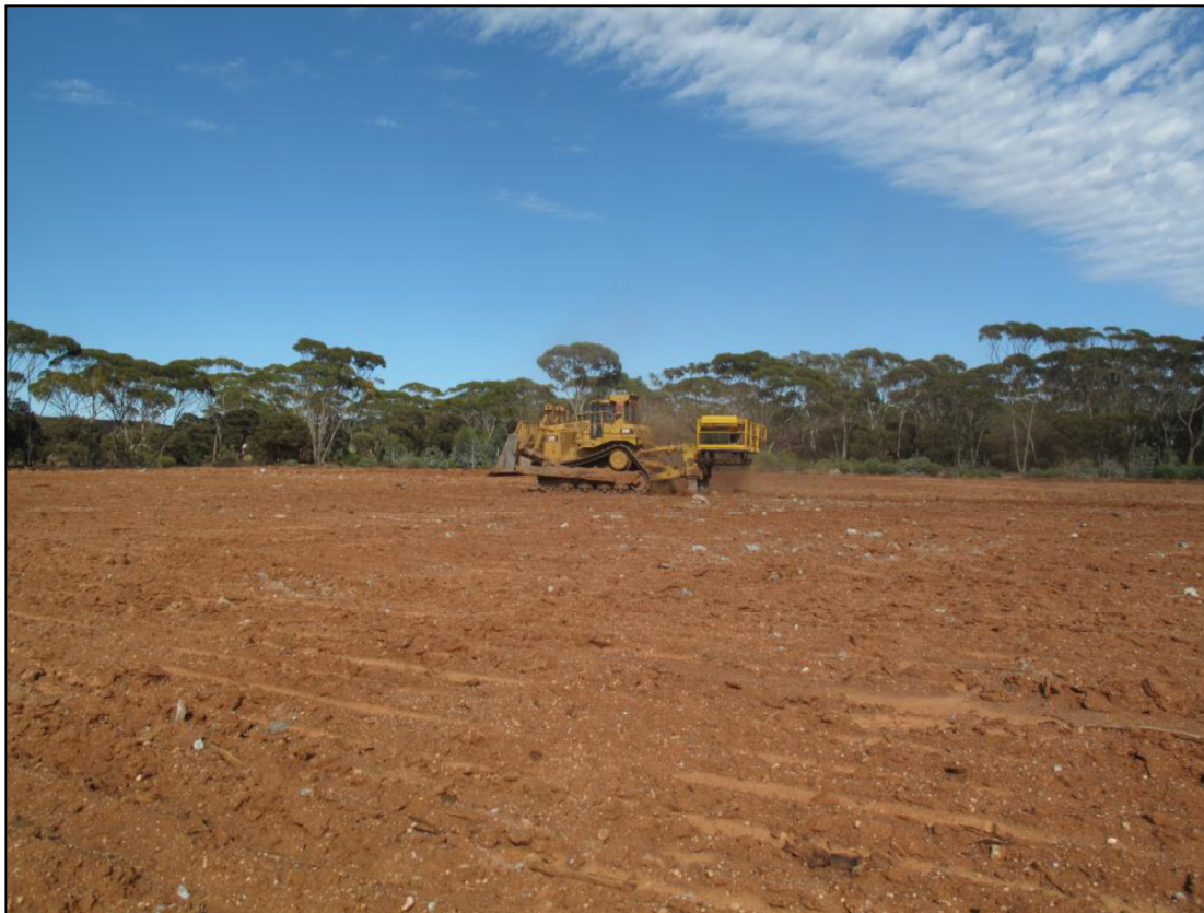
Figure 2: Ripping and seeding at Wattle Dam as part of rehabilitation works
