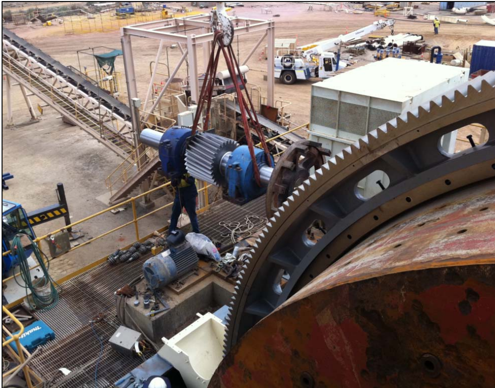
Figure 3: SAG mill girth gear refurbishment
