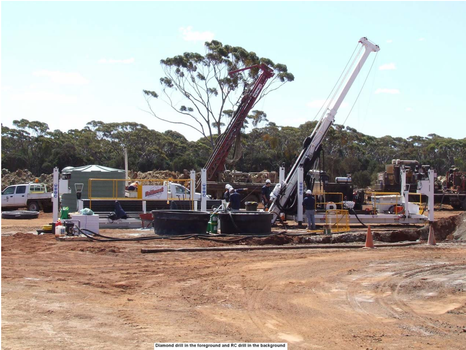
Diamond drill in the foreground and RC drill in the background
