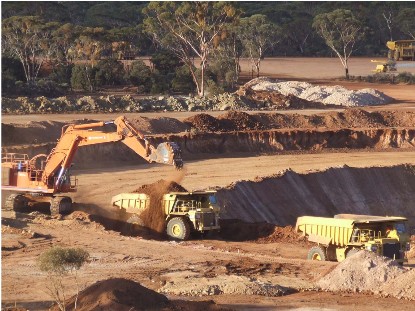
Progressing the Cut Back at Wattle Dam Gold Mine
