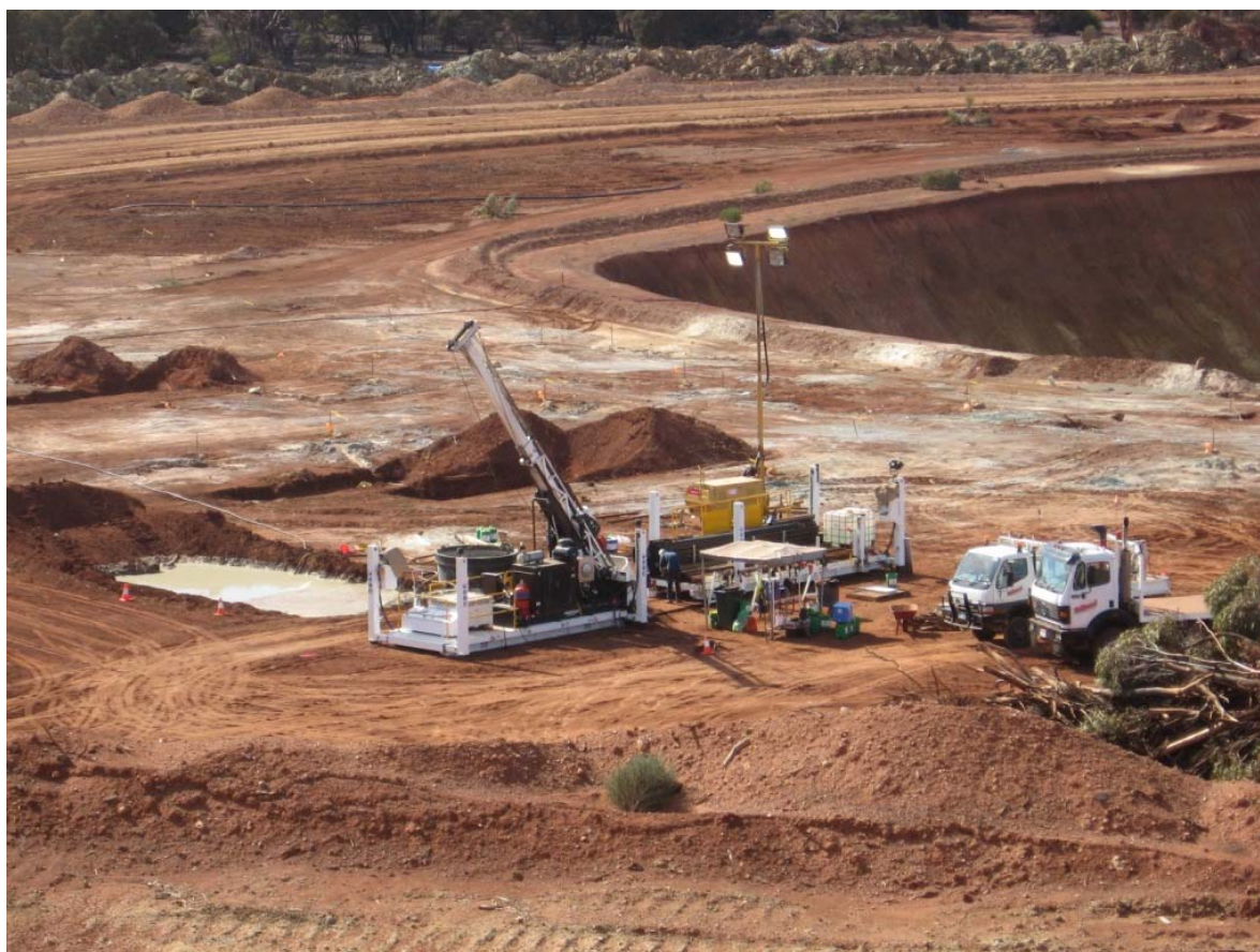
Diamond drilling beneath the Wattle Dam pit
