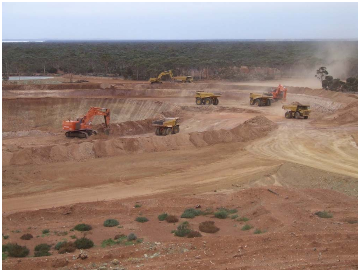
Commencement of Cutback of Pit at Wattle Dam
