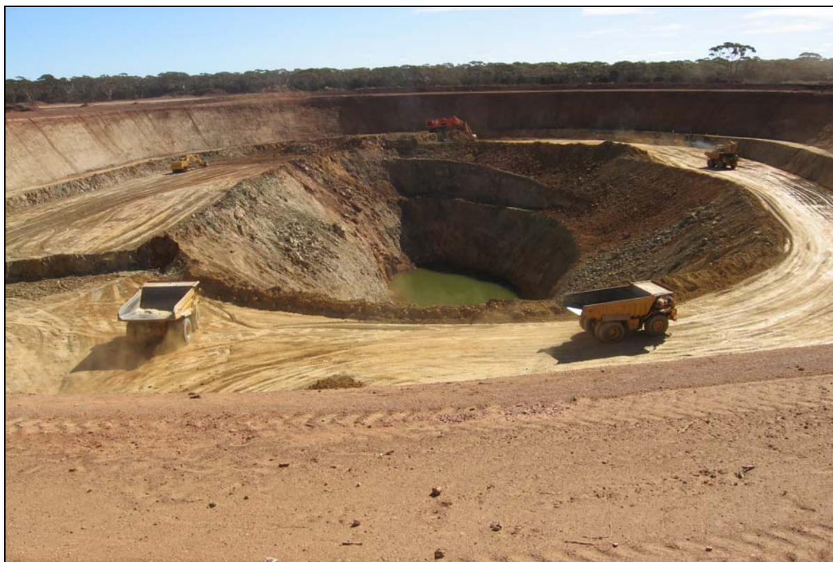
Open Pit Cut Back in August 2008
