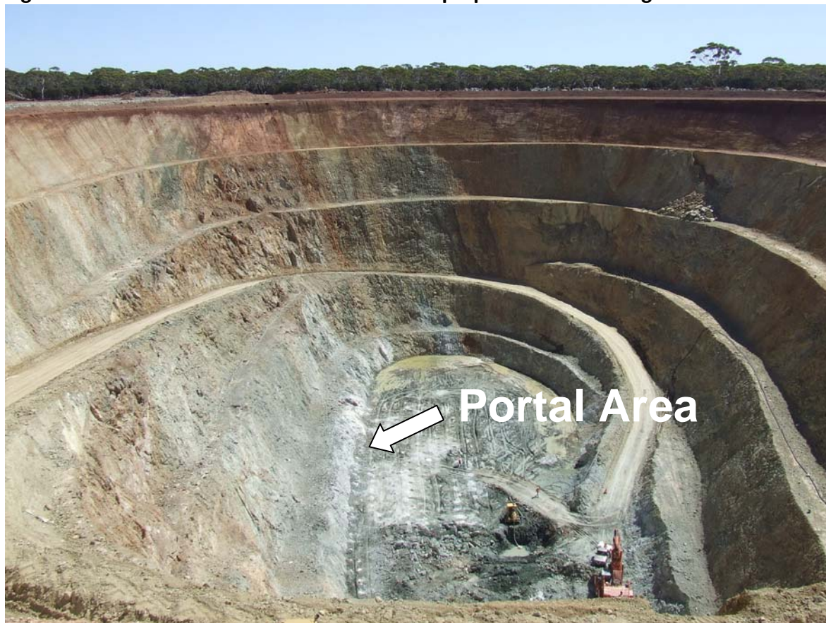
Fig 1: Cut Back Pit in March 2009 where Portal preparations have begun
