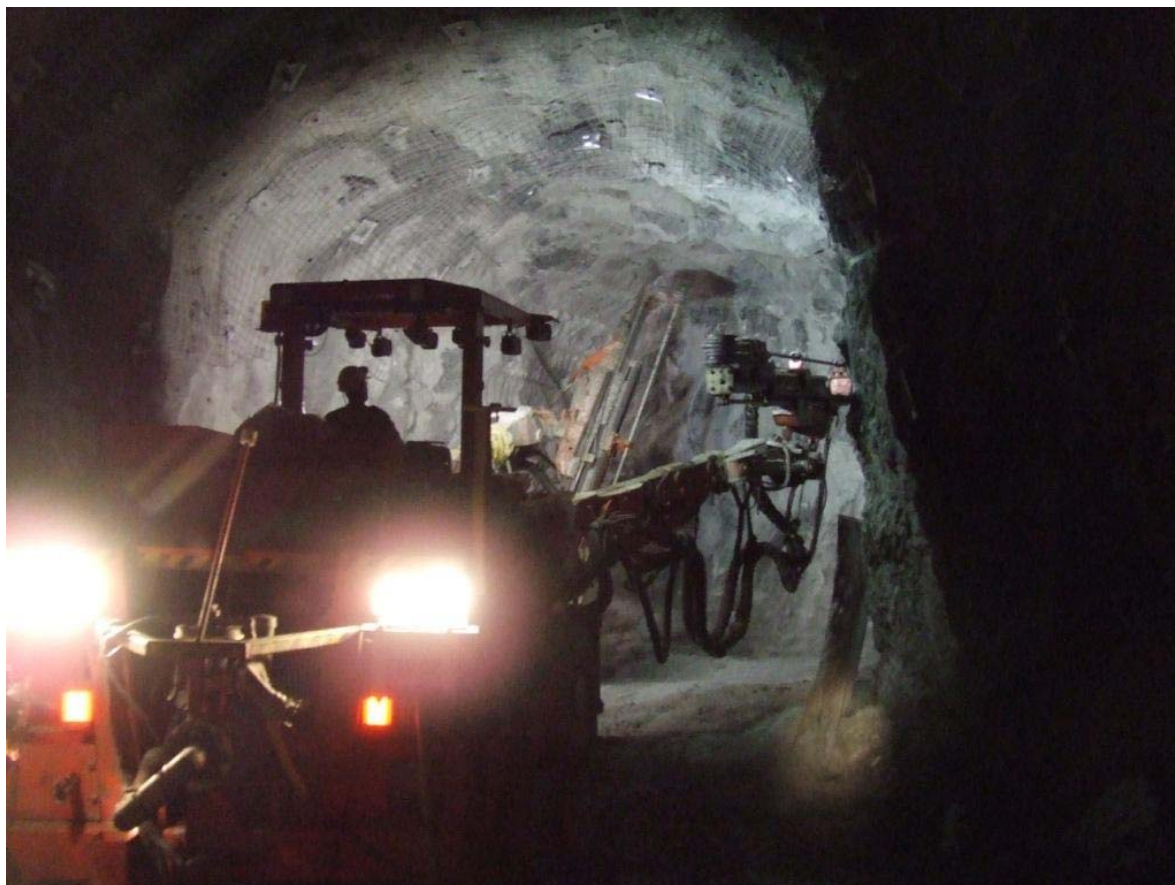
Picture: Decline work at Wattle Dam
